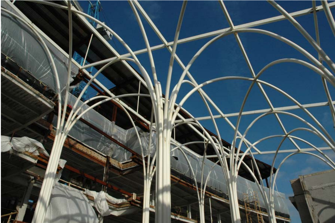
Steel Framing for Atrium Skylight Glass
