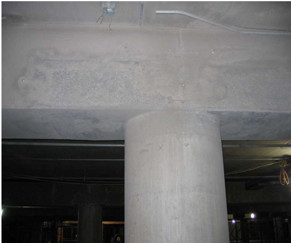
Garage Beam Repair
