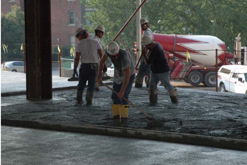
Crews Level Newly Poured Concrete Floor
