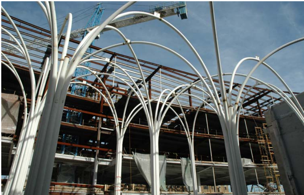
View of the Atrium Arches from Cret Building
