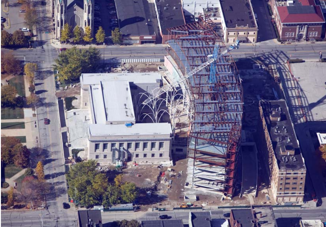
Aerial View of Central Library Construction Site
