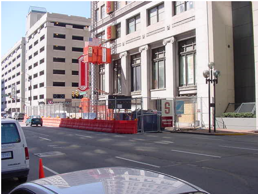
Man-Material Lift Used During Renovation of Fletcher Building in Downtown Indianapolis
