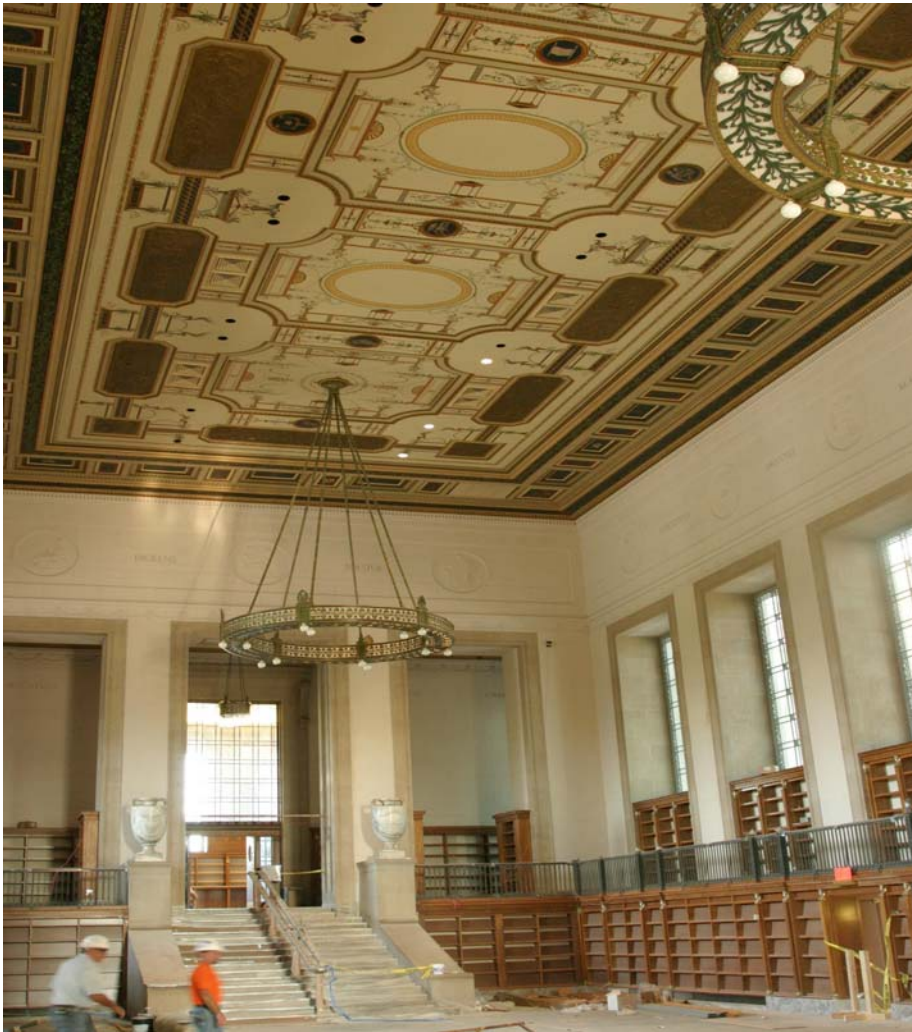
Restored Ceiling and chandelier in the Historic Cret building
